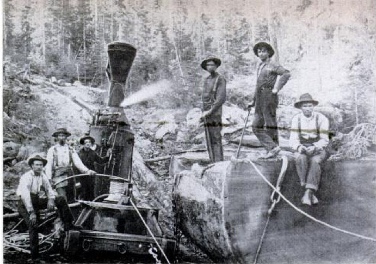
Donkey steam engine was the workhorse. Mounted on skids, it reeled in cable to pull itself up the mountains
